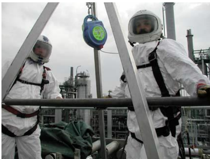
Figure 5: Example of life support system (LSS) organisation for inert entry on the top of a reactor.
