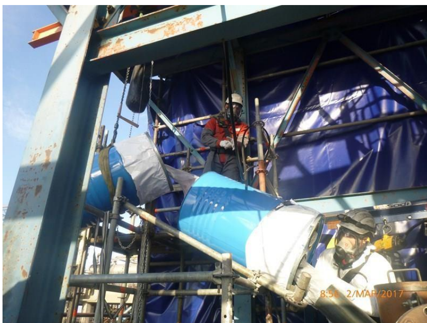
Figure 12: Drum emptying in a difficult location with dust containment. The opening of the drum is enclosed in a sleeve to prevent any dust formation.
