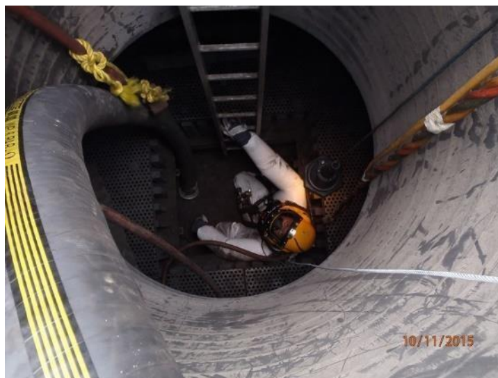
Figure 8: Working in catalyst reactor with life support system.
